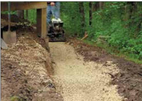
1. Prepare the Site
